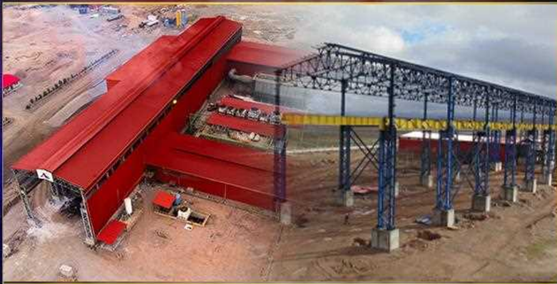
Industrial Shed Construction
